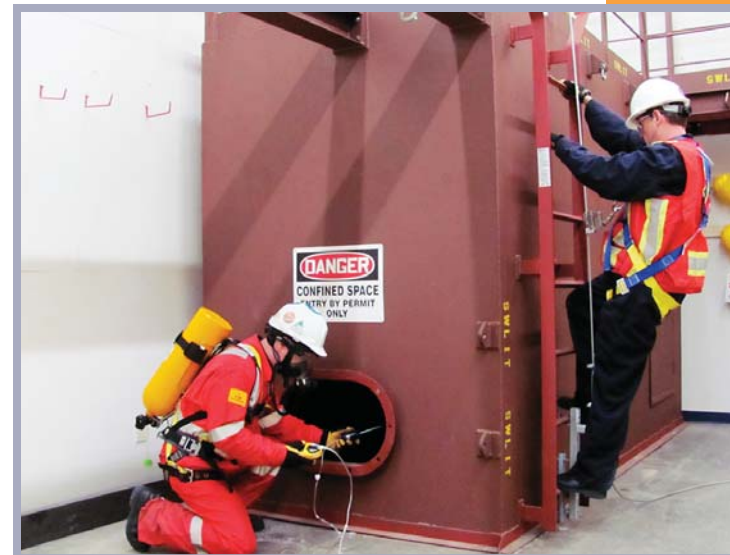
Person kneeling is demonstrating gas detection; at right ladder climbing device which is a component of fall protection demonstration.
